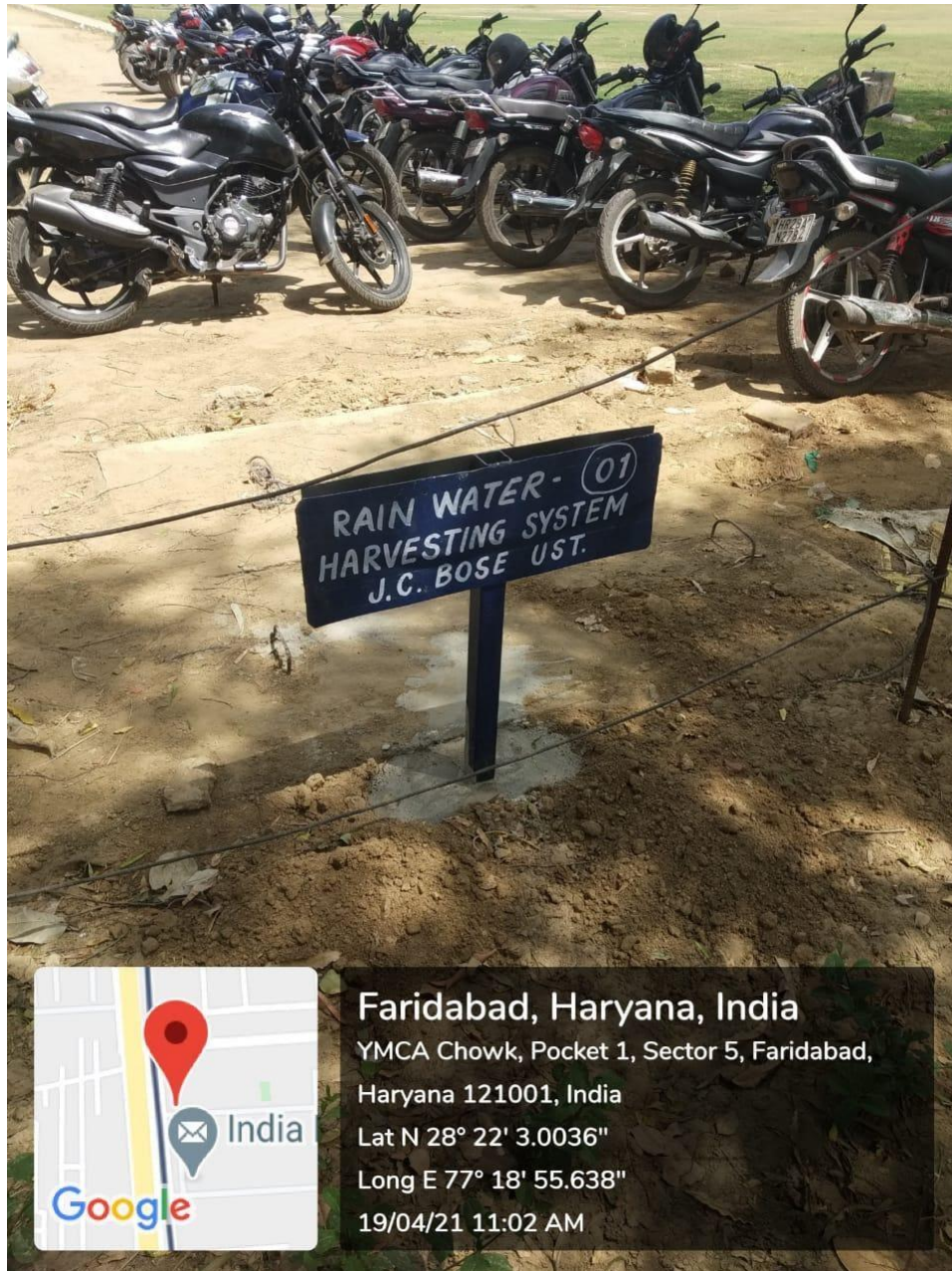
Image-05: Rainwater harvesting structure in playground near Main Parking area
