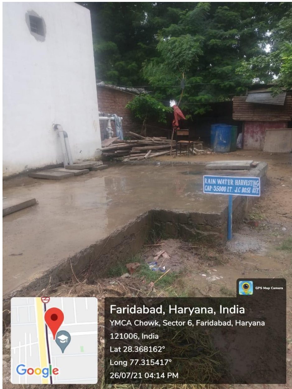
Image-09: Constructed tank corner of Playground area
