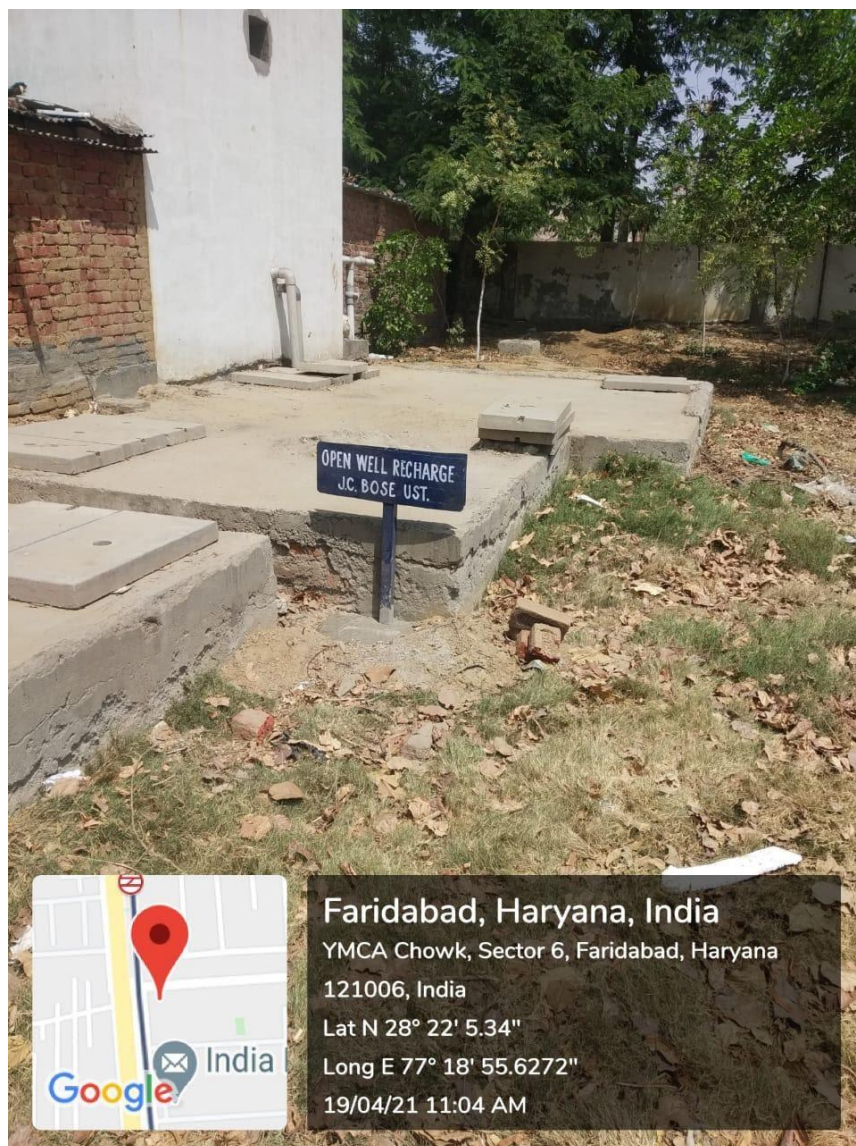
Image-06: Recharge Well at rear corner of Playground area
