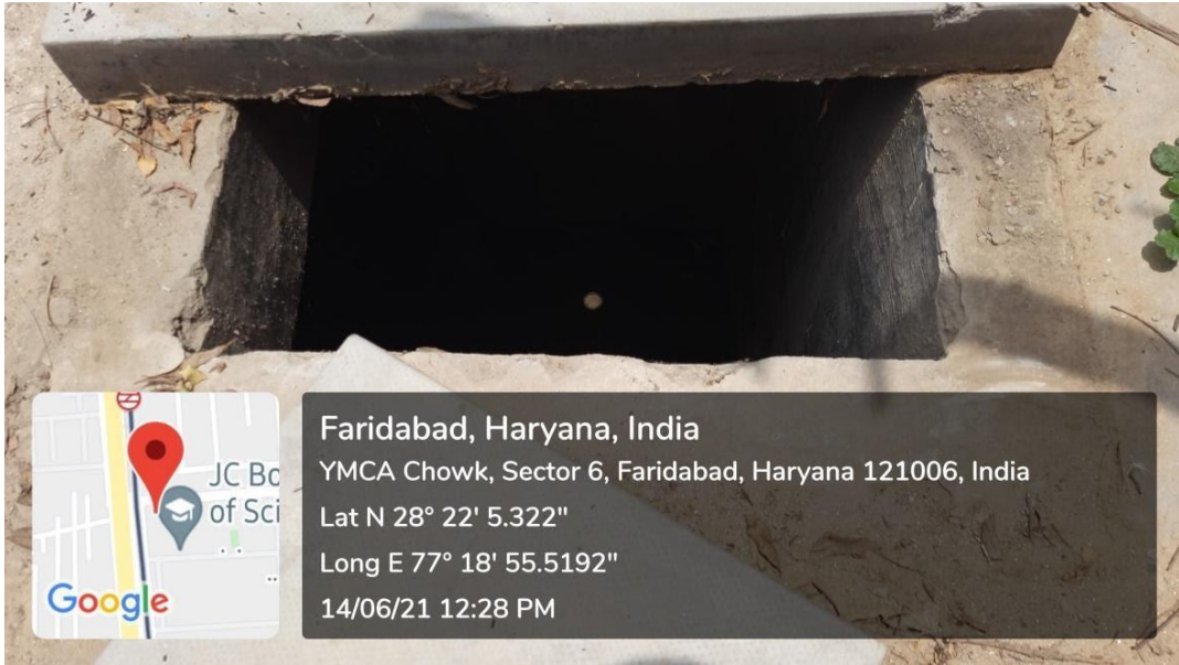
Image-07: Recharge Well at rear corner of Playground area
