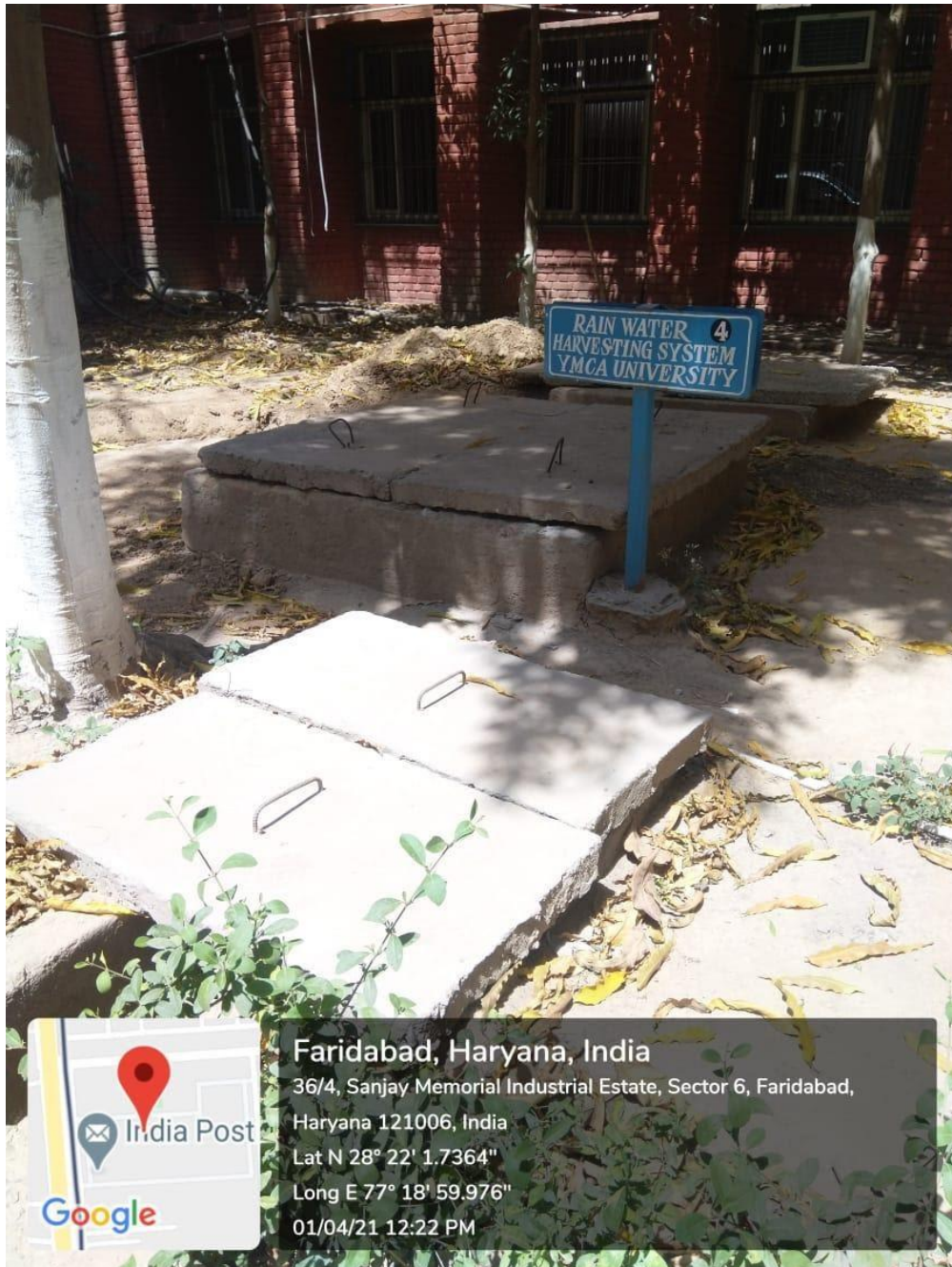
Image-03: Rainwater harvesting structure at back side of Shakuntlam Hall
