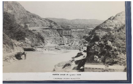
Concreting operation started 1956
