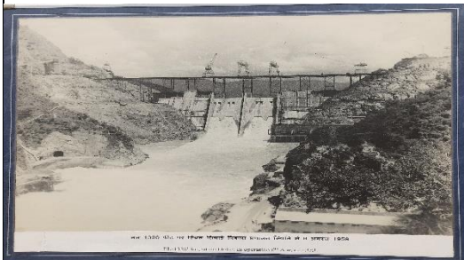
EL'1320 Irrigation Outlet in Operation 6 th august 1959
