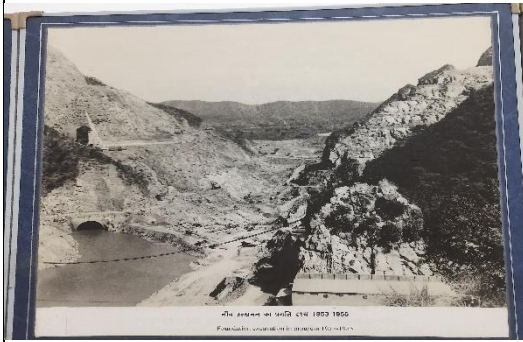
Foundation excavation progress (1953-1955)
