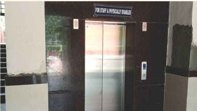
INSTALLATION OF LIFT
